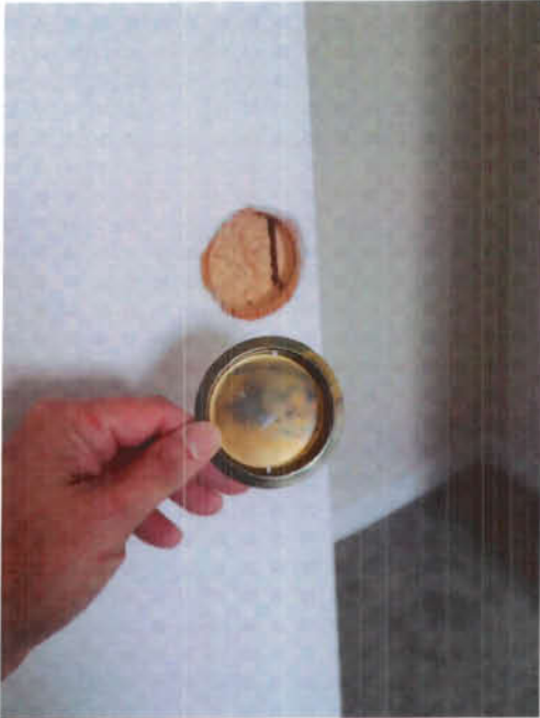
Qaiser left on the attached brass hardware when painting, despite it not being attached to the door.
