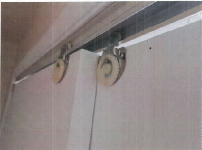
Qaiser improperly installed these closed doors, and now cannot fully open or close.
