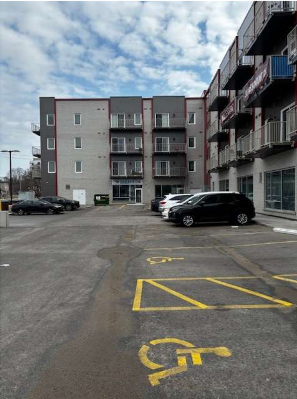
Dental unit – sign is up but the unit is still incomplete & under construction. Nobody working on the unit when we were there
