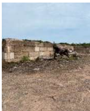
Yard Storage Blocks
