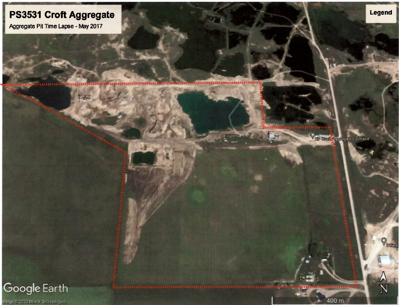
Figure 2: Satellite image of site taken in May of 2017 showing excavation beginning in the northwest corner of the southern land package.
