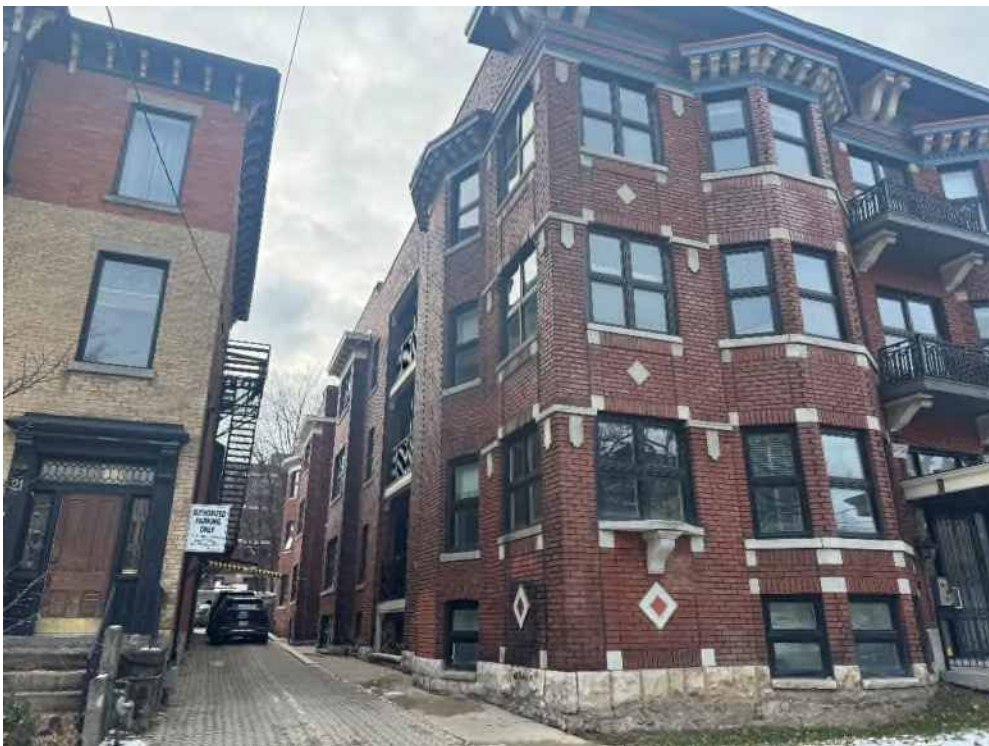
East side of the building
