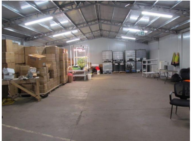
Open Portion of Office Structure
