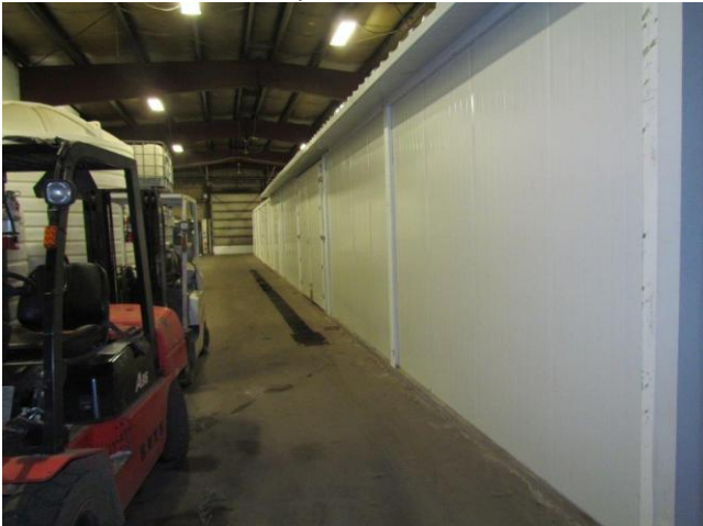
Office Structure & Shop Area
