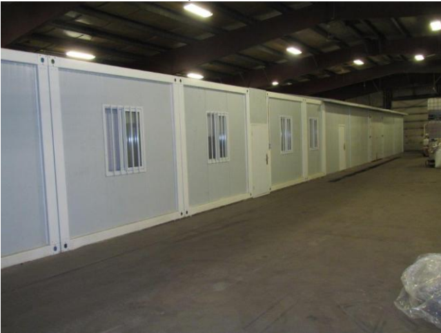
Office Structure in Shop
