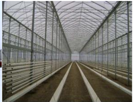
Photo of greenhouse complex - Interior view
